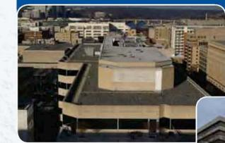
**2000 Pennsylvania Ave, Washington, DC:** Removed existing urethane IRMA roof and installed hot rubberized asphalt on lower roofs, main roof and penthouse.
